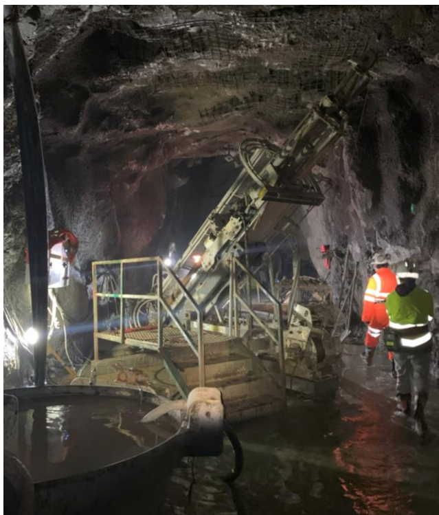
Figure 10.2: Underground Drill Rig at the Kearney Vein
