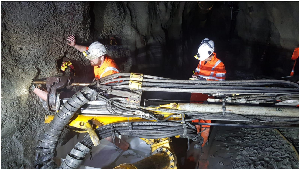
FIGURE A: drilling a probe hole.
