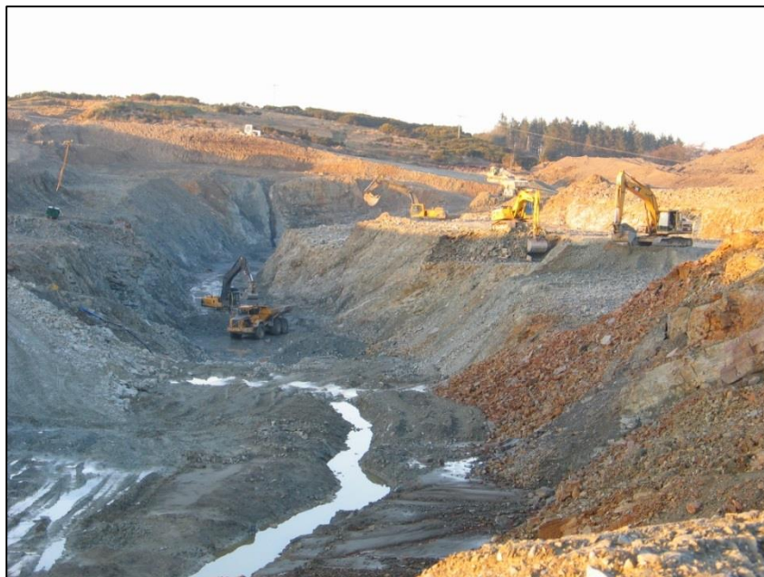
FIGURE 8: KEARNEY VEIN EXCAVATION IN FEBRUARY 2008
